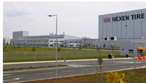
Nexen Tire production plant, Czech Republic
