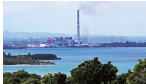
Thermal power plant Felton, Cuba
