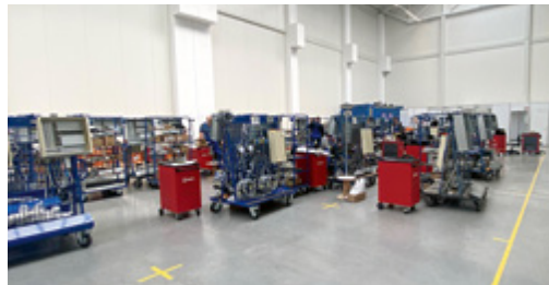
Assembly hall of switchboards for Schindler escalators
