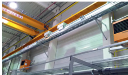
Hall FELS in Ilava
