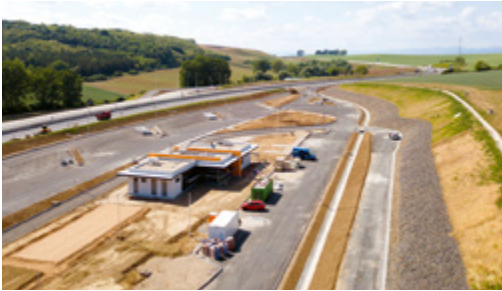
Rest area on highway R4 Košice – Milhošť
