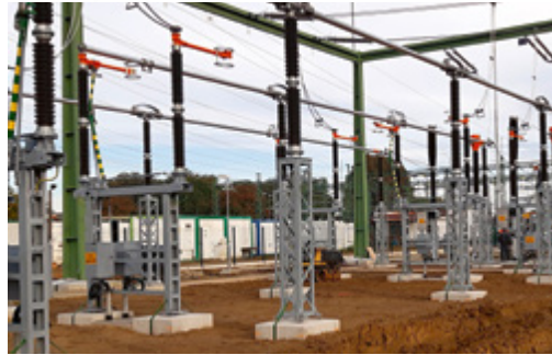
Construction of 245 kV ES Opočíněk
