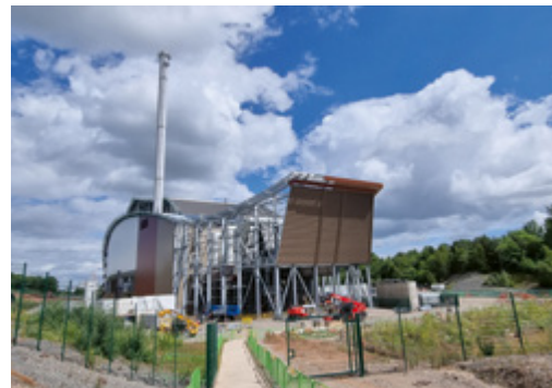
Incinerator Newhurst, Great Britain
