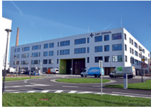
New Generation Hospital in Michalovce
