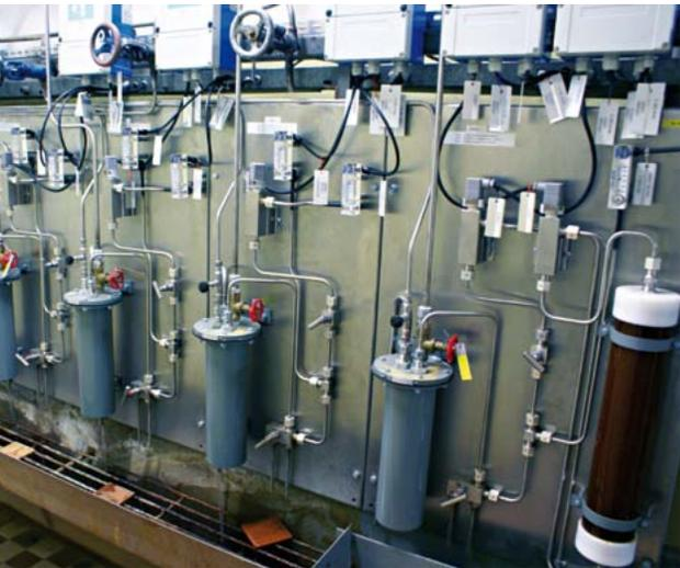
Panel for pressure and temperature adjustment of the samples in power engineering
